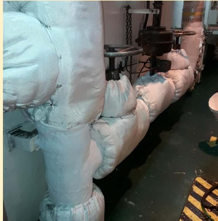
THERMAL INSULATION PILLOWS AT PIPE NETWORK
