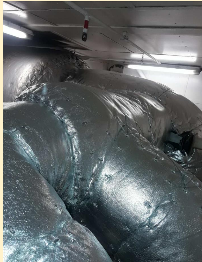
THERMAL INSULATION PILLOWS (HIGH TEMPERATURE)
