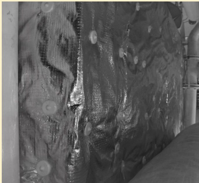
THERMAL INSULATION OF SILENCER
