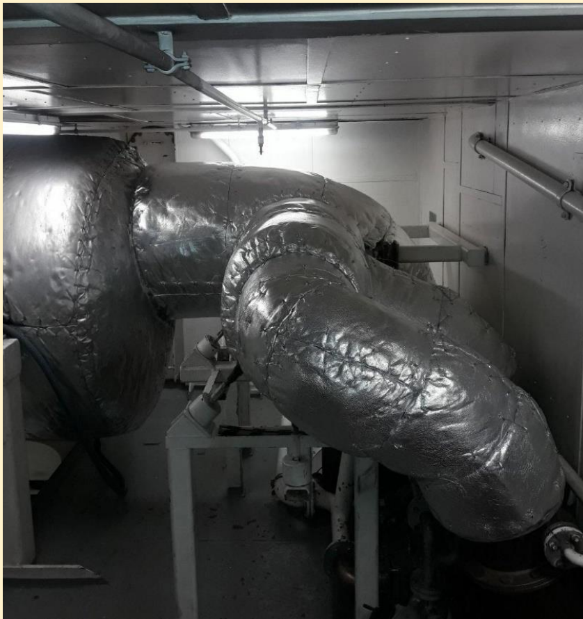
THERMAL INSULATION PILLOWS (HIGH TEMPERATURE)
