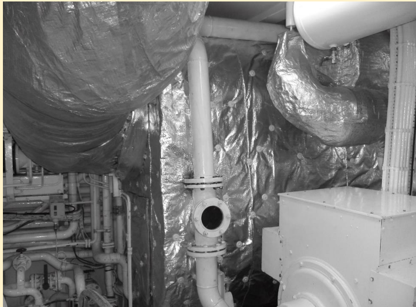
THERMAL INSULATION OF SILENCER
