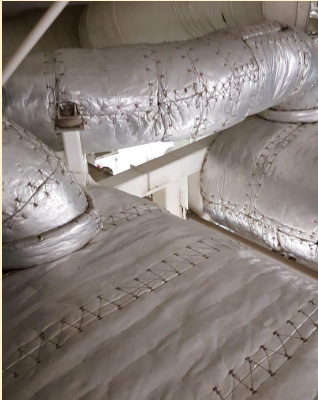
THERMAL INSULATION PILLOWS (HIGH TEMPERATURE)
