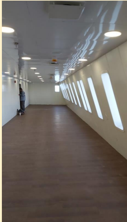
VINYL TILES IN WOOD IMITATION COLOUR FOR AIRSEAT/DECK
