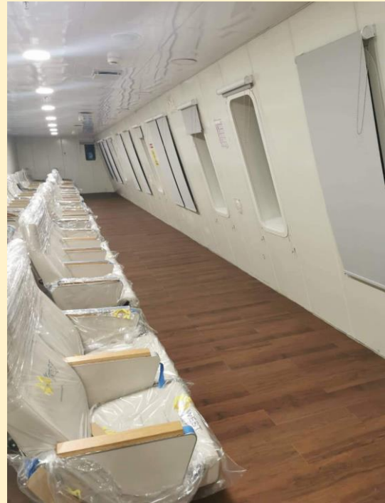
VINYL TILES IN WOOD IMITATION COLOUR FOR AIRSEAT/DECK
