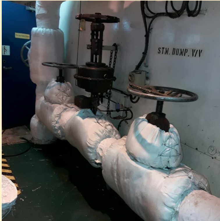
THERMAL INSULATION PILLOWS AT PIPE NETWORK
